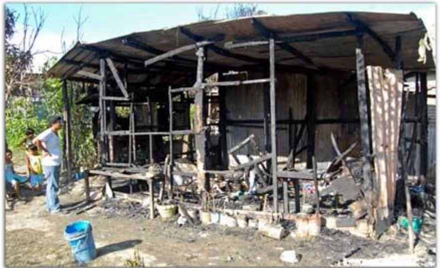
Pastor Ogie's house was completely destroyed in the fire.
