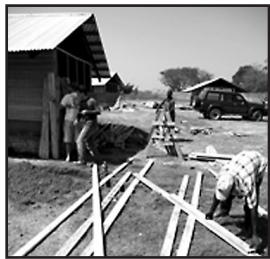
Construction continues on the Cijanano campground and ministry center
